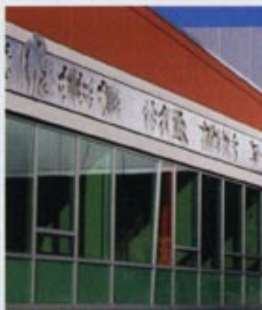
The Beecher School, in New Haven, CT, is wrapped by a 500-foot ornamental aluminum frieze.
